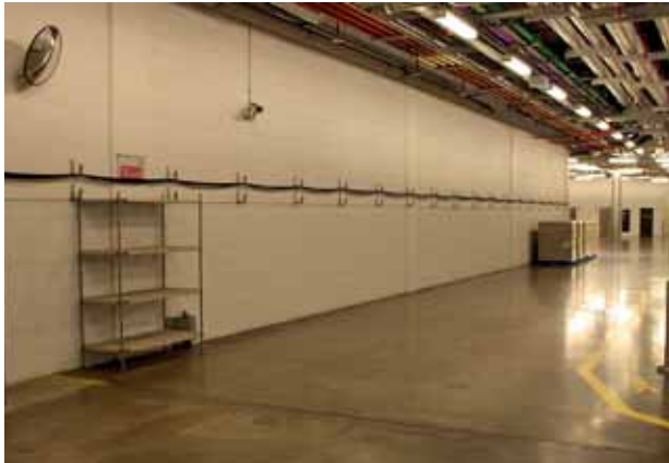
Cable hooks from loading dock and Level 3 OB riser (banquet OB cable run).
